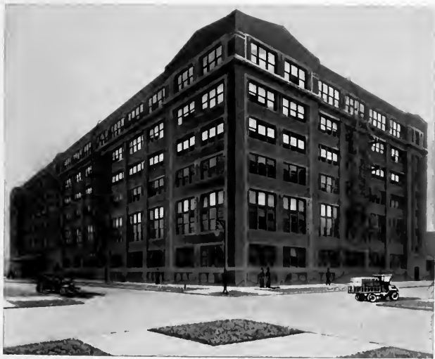
The Grocery Building, constructed of steel ribbed concrete. Seven acres of floor space
